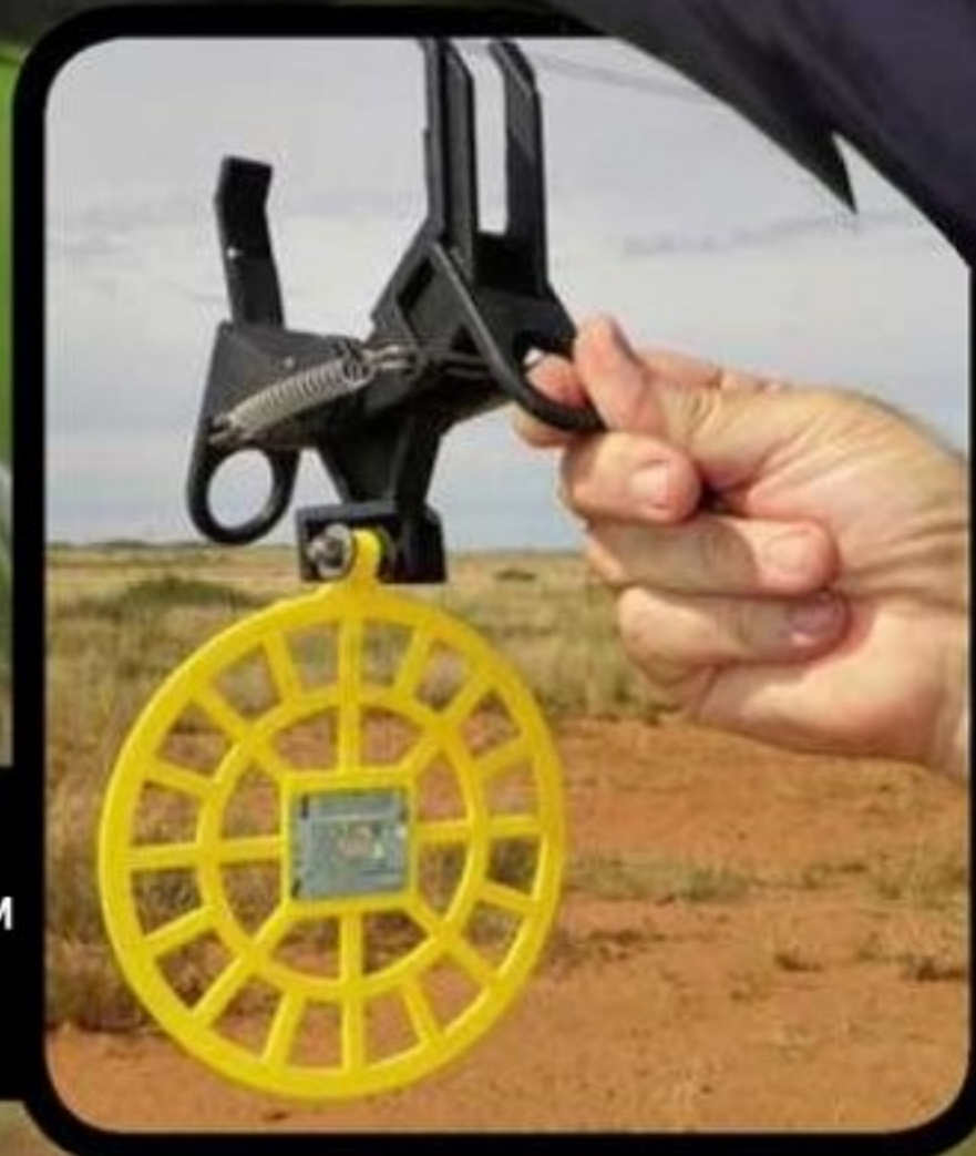
THESE FLAPPERS ON POWER LINES HELP BIRDS TO SEE THE DEADLY WIRES AND AVOID THEM WHEN THEY SWOOP DOWN TO LAND IN THE WHEAT FIELDS OF THE OVERBERG.
